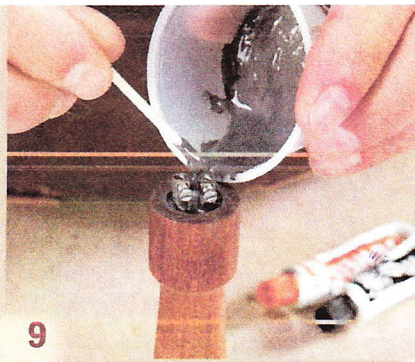
9 Cement the terminals in place with J-B Weld. This adhesive can withstand high heat and doesn't conduct electricity.
